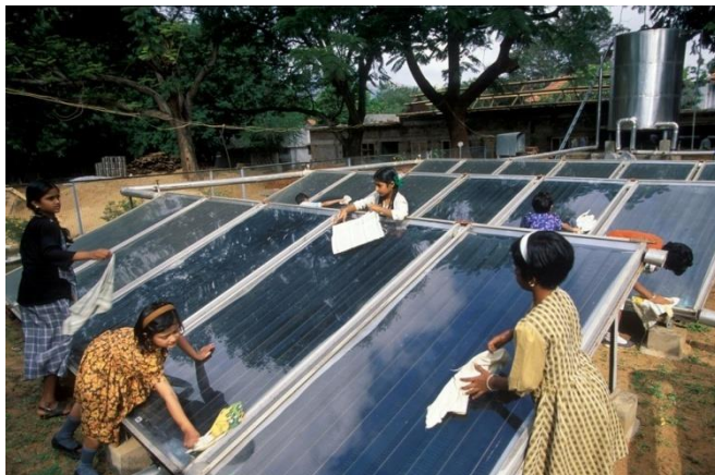
Solar hot water heating - India
