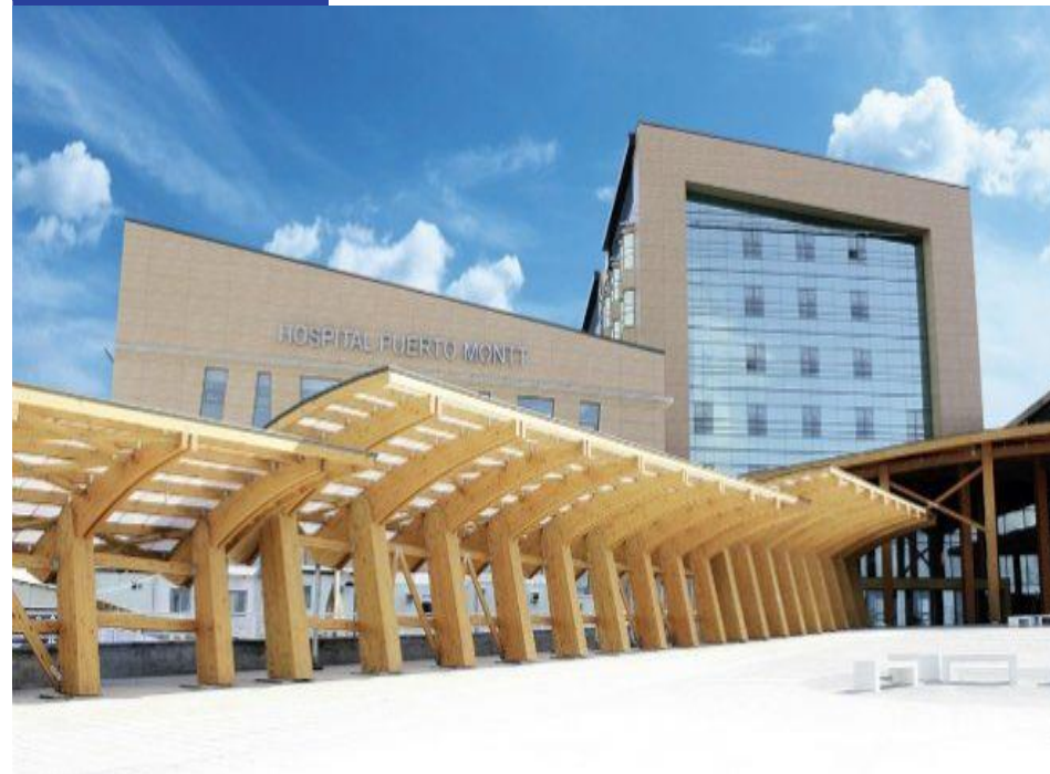
HOSPITAL BASE DE PUERTO MONTT
