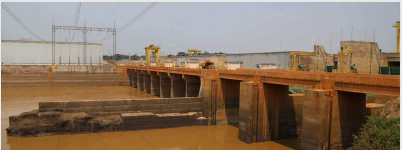
Jirau hydroelectric dam, Porto Velho - Rondônia, Brazil. Photo Credit: PAHO.
