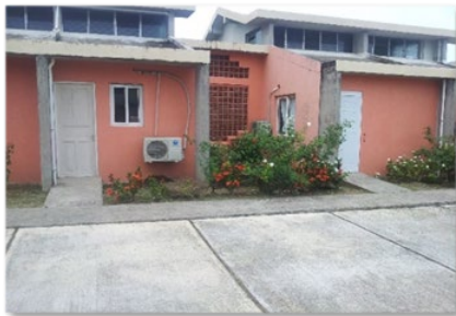
Image 8: 'Before retrofitting' – glass louvres, vent blocks, wood doors
