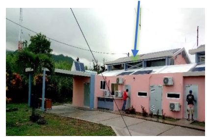
Image 10: 'After retrofitting' – Hurricane rated windows and doors installed
