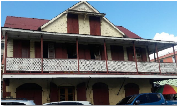
Image 6: Wood Colonial Shutters, Dominica, post-Hurricane Maria
