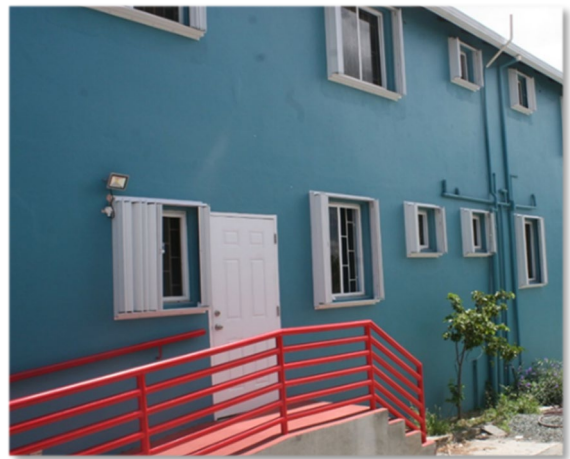
Image 4: Accordion shutters installed at facility
