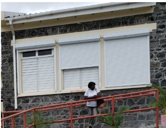
Image 18: Shutters in various stages of open and fully closed
