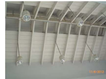
Main entry ceiling
