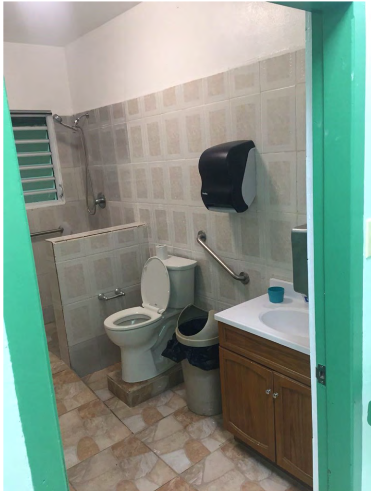
Photograph 22 New Upgraded Bathroom
