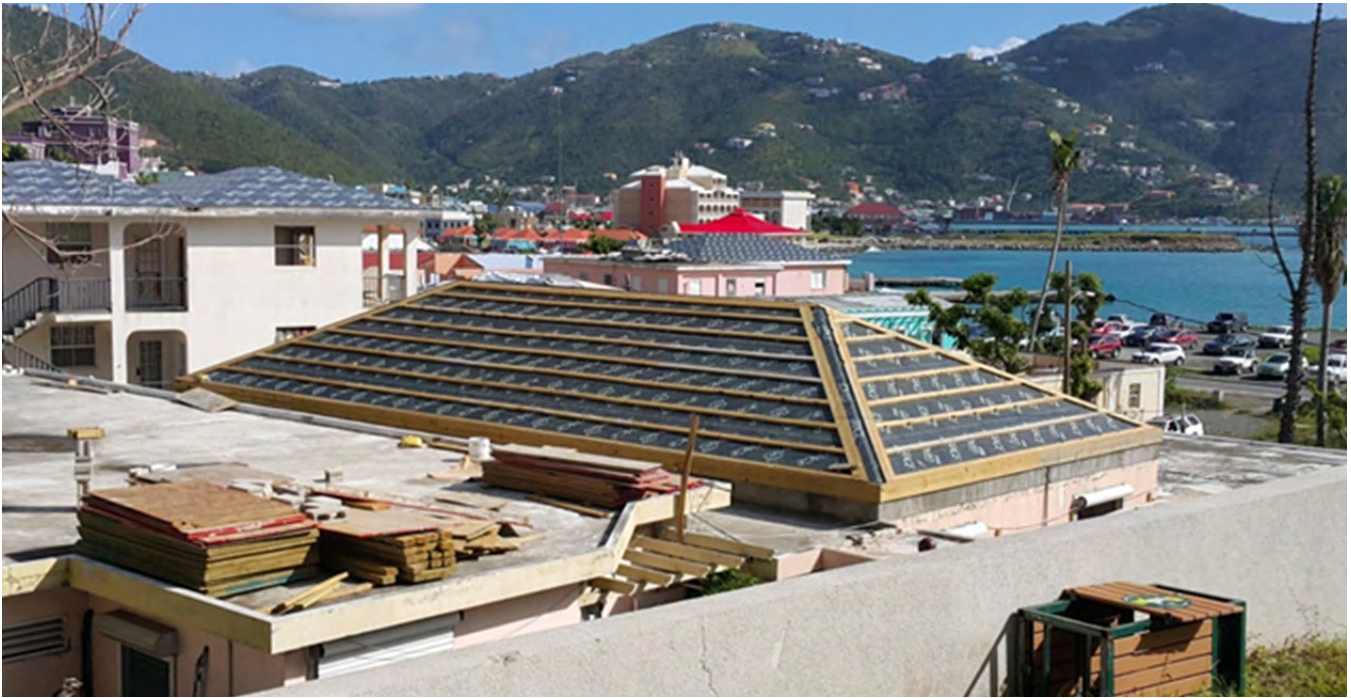
Photograph 12 Roof Under Renovation
