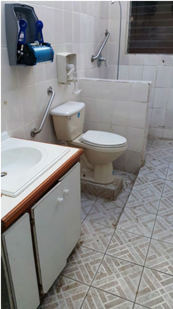
Photograph 21 Typical View of Old Bathroom
