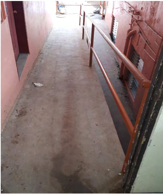
Photograph 8 Old Open Ramp
