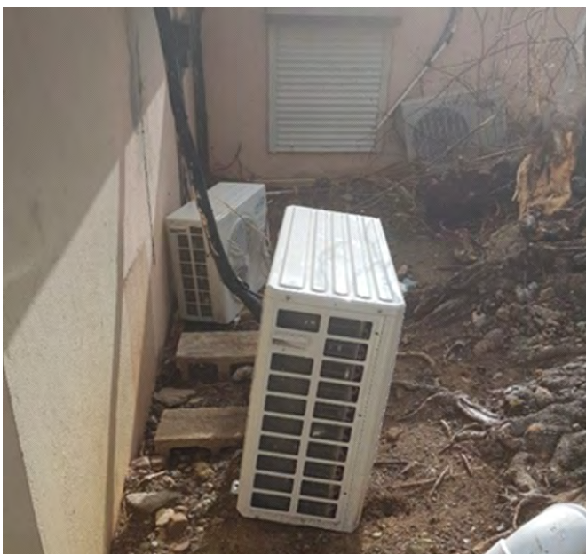
Photograph 6 Dislodged Condenser
