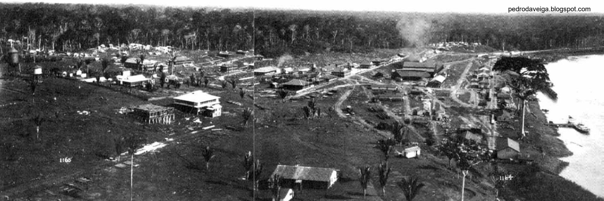
Madeira Mamoré railroad construction in Porto Velho - Rondonia - Brazil
