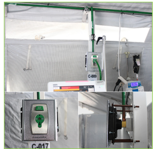
Image 10: Indoor oxygen intakes (EMT SARI MoH Ecuador).
