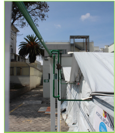
Image 1: Oxygen facilities in a SARI EMT (EMT SARI MoH Ecuador).
