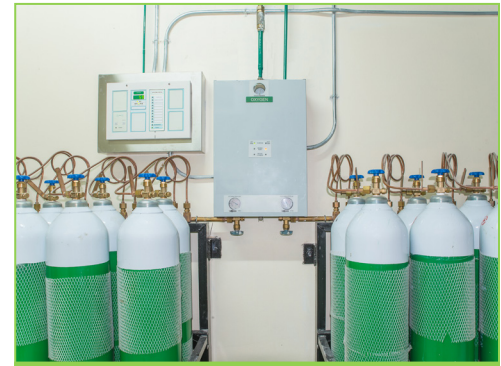
Imagen 7: Group of cylinders connected through a manifold.
