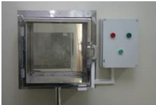
Pass through, for entry / exit of material that can not be autoclaved
