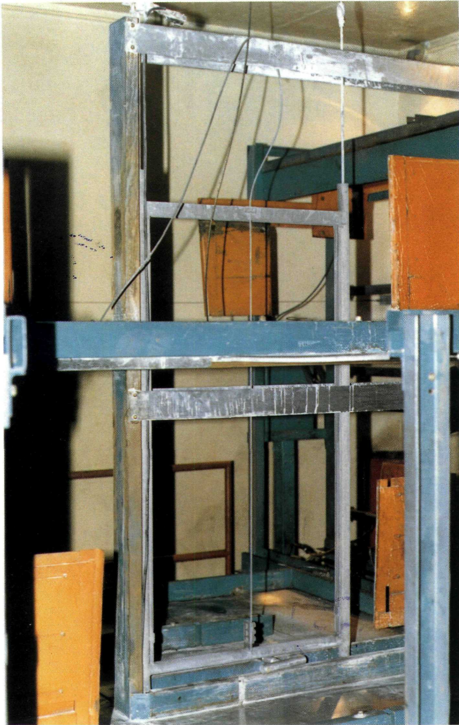
13. The empty source rack and the entangled source hoist cable.
