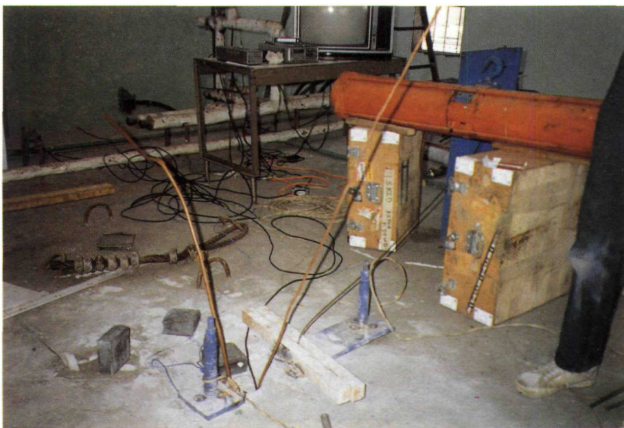
12. The radiation room roof during securing of the sources.
