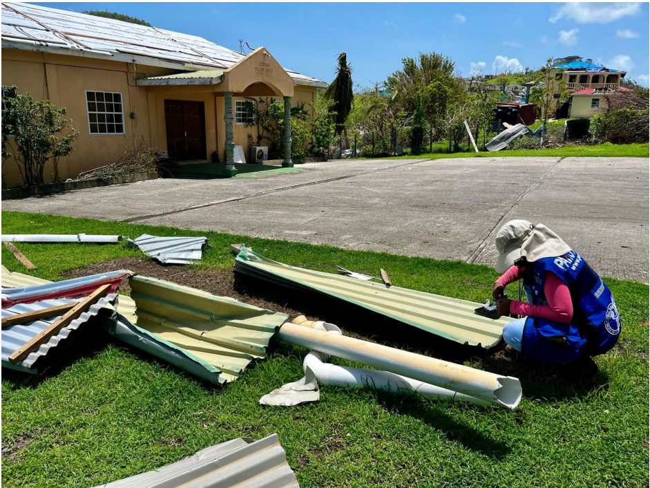
Inspection of galvanized roof sheets in L'esterre Health Centre, Carriacou
