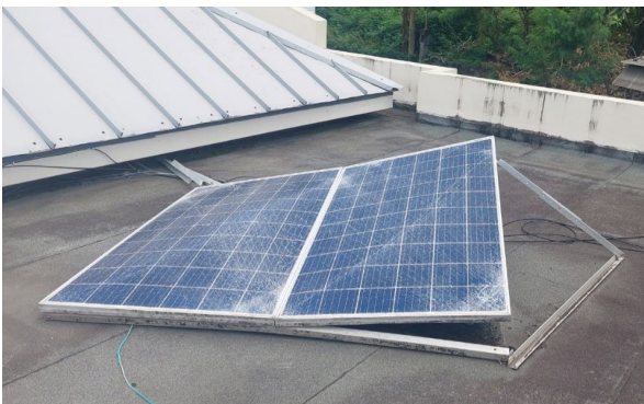
Damaged solar panels – Buccament polyclinic
