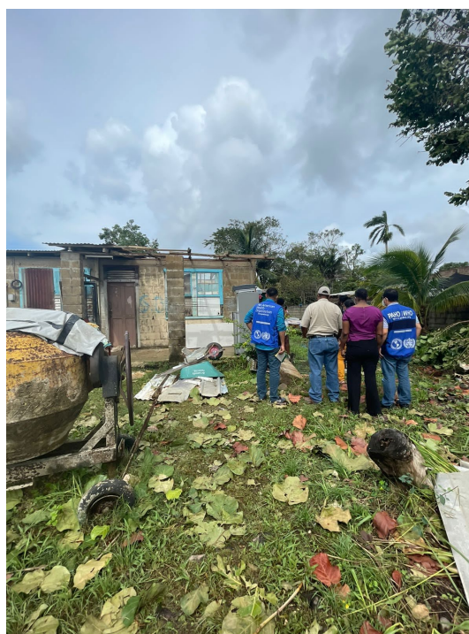
4 Nov. 2022: Inspection of damaged homes in Hattieville, Rural Belize District
